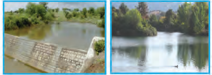
Fig : 11 Check dam Percolation pond
