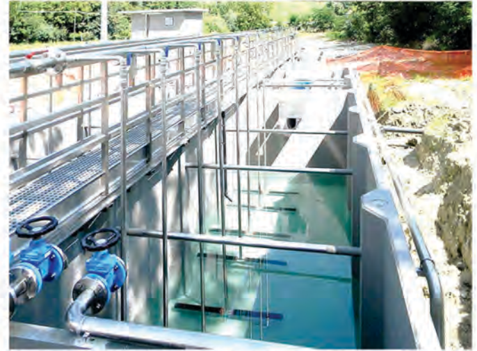
Fig 4: Extended Aeration System
